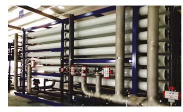
Fitran UF prefiltration equipment provides reliable protection for UF and other membranes. Reduce particle loading to membrane systems with no interruption to system flow.
